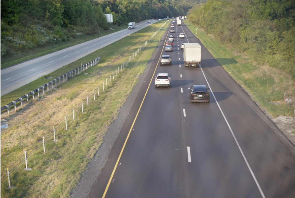
UTBWC used to Seal and Level Concrete followed by a Structural 2 inch SMA Overlay I-78, Lehigh County
