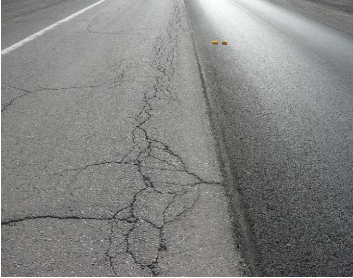
Fatigue, Longitudinal & Transverse Cracking – Moderate
