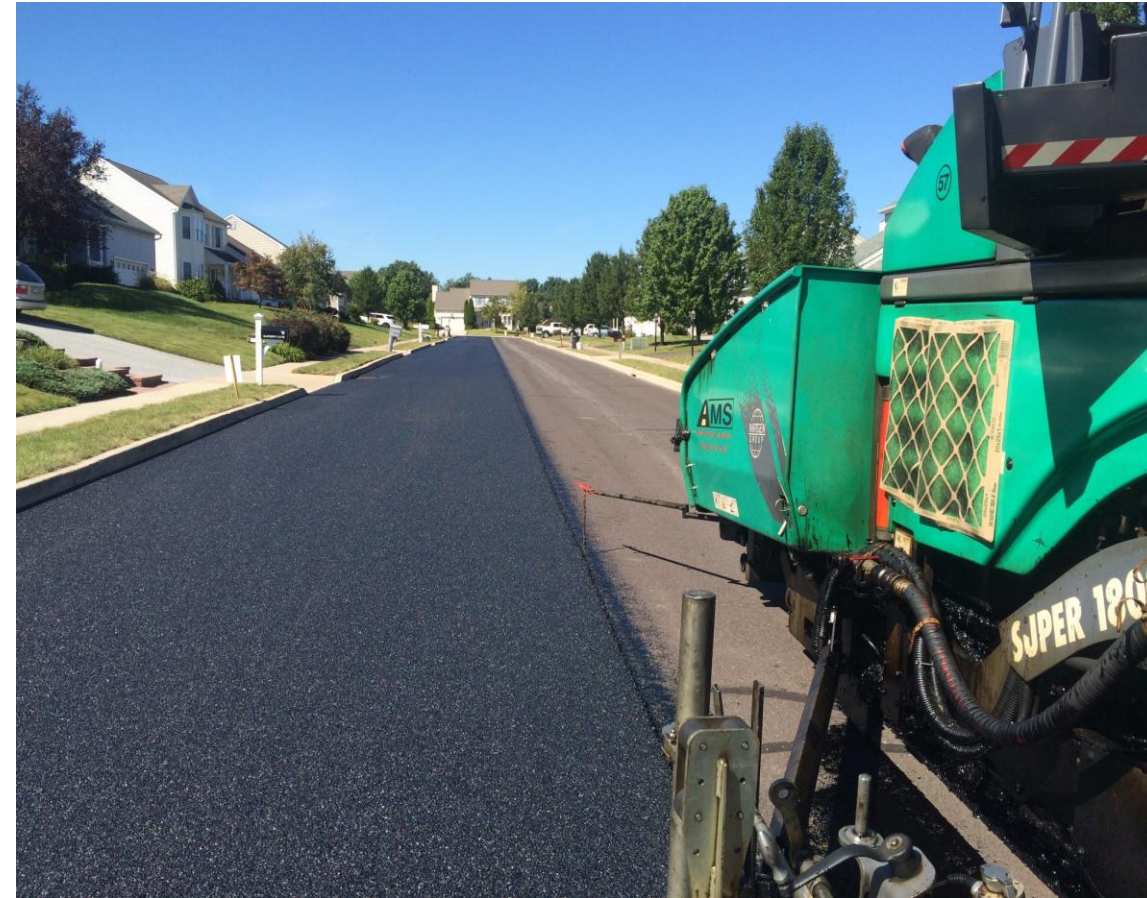
UTBWC Gradation B Residential Development
