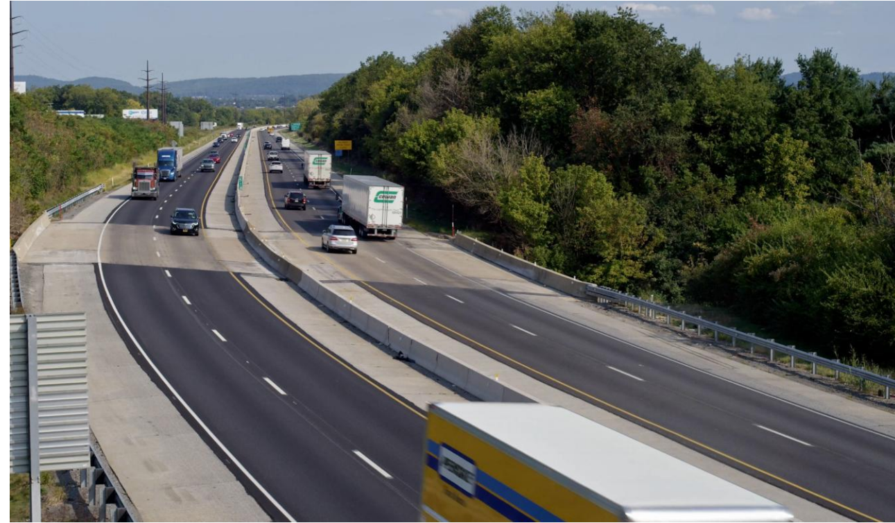
UTBWC used as final surface over Concrete I-78 Lehigh County
