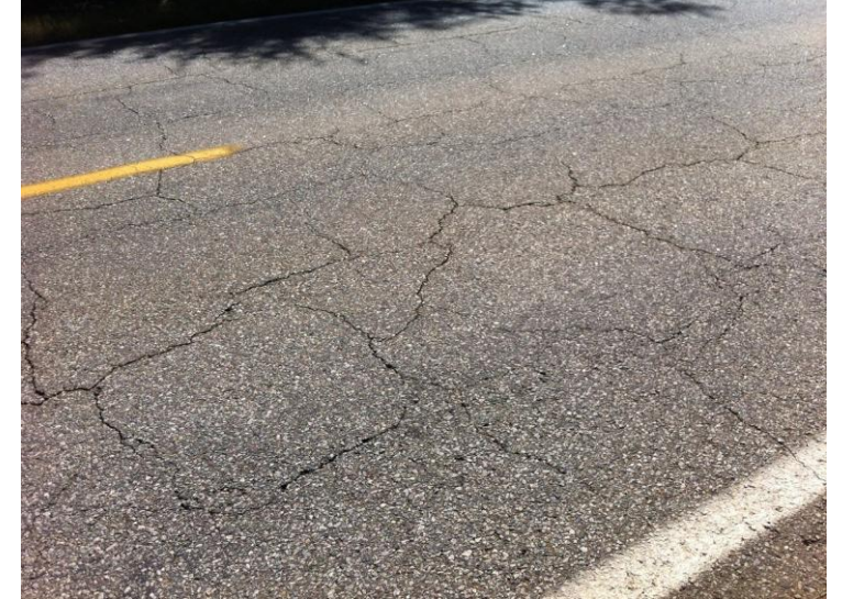
Block Cracking
