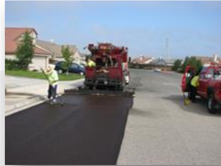
Unacceptable transverse joint
