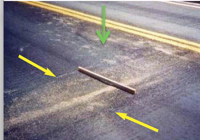
Unacceptable transverse joint
