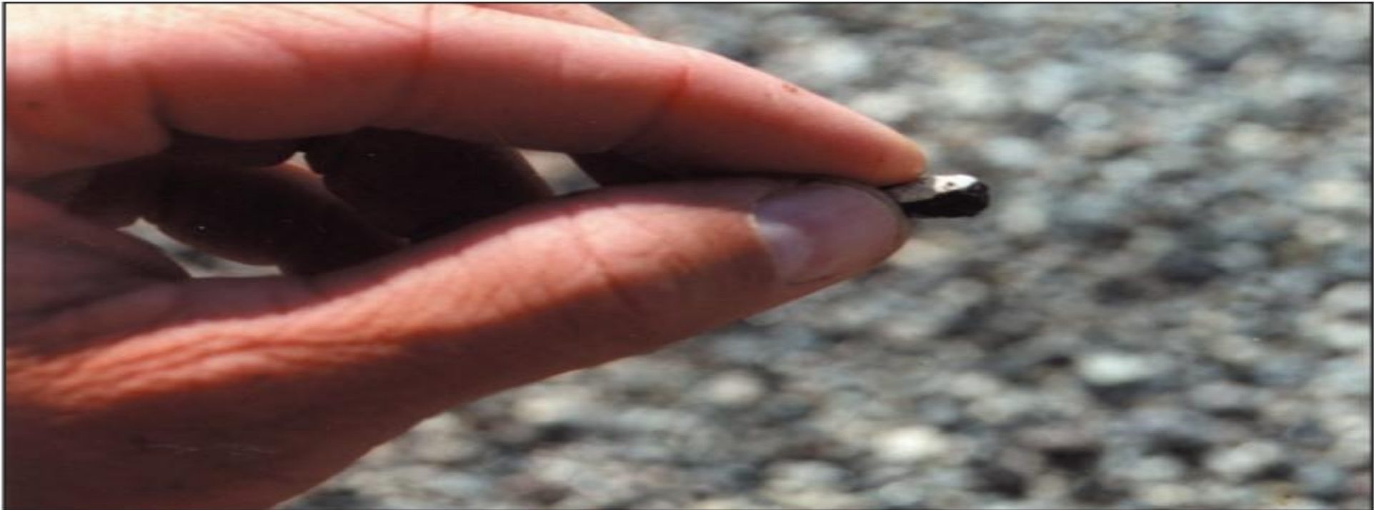
Figure 4.4. Proper embedment (~70%) into the residual asphalt
